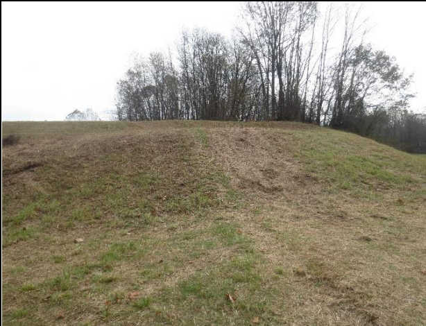
Image 33: ASW training dike slope. Note vehicle path and bare areas
