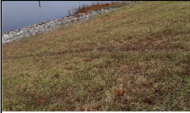
Image 3: Worn path from crest to Normal Pool Elevation
