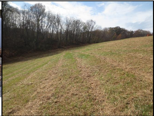
Image 8: Downstream slope from left groin
