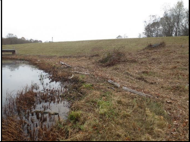
Image 32: Woody debris and logs along ASW inlet
