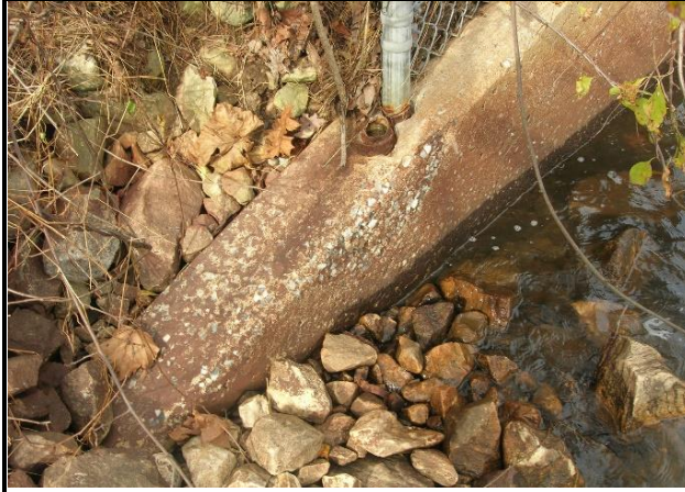
Image 27: Pitting in right impact basin wingwall
