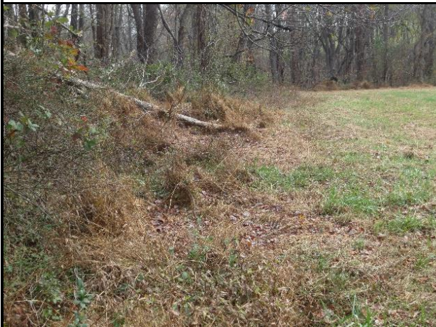
Image 41: ASW inside slope, training dike facing downstream. Note trees within 15 feet of channel
