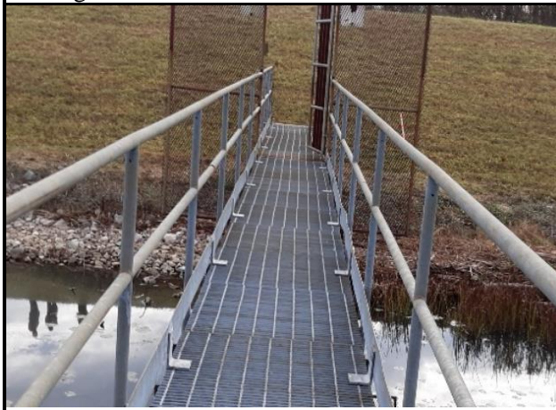
Image 45: Catwalk leading to intake tower
