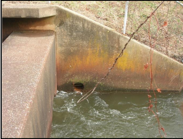
Image 25: Left toe drain outlet at impact basin
