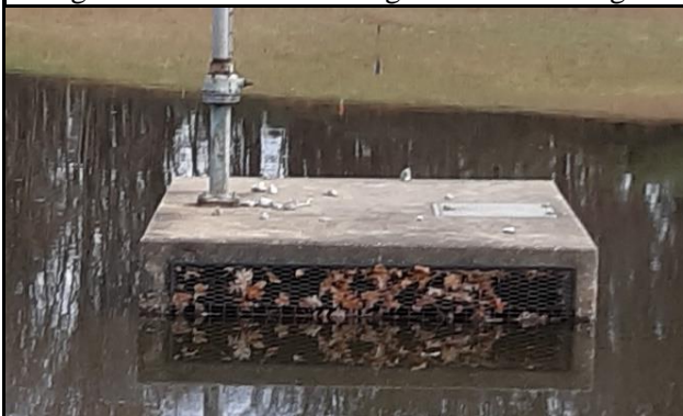
Image 17: Leaves collected on PSW riser trash rack
