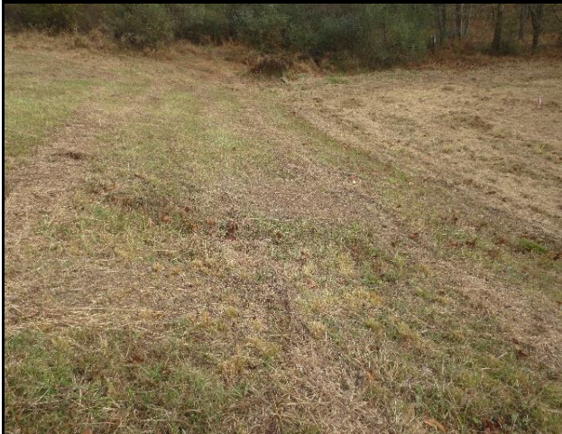
Image 9: Depression in downstream slope near toe
