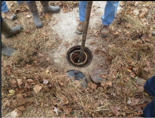
Image 51: Rate control piping butterfly valve operation
