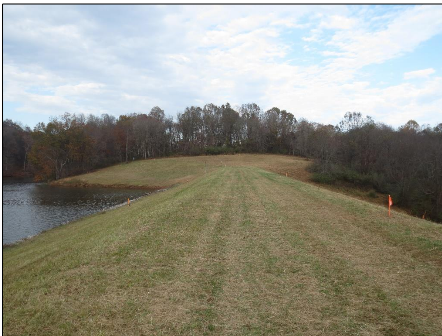
Photograph 1: Dam crest looking towards left abutment.
