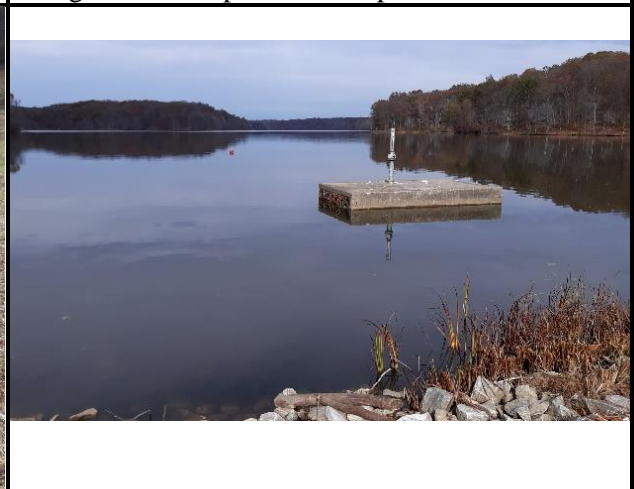
Image 16: Downstream face of PSW riser
