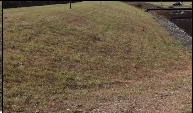
Image 4: Upstream slope from left groin. Note depression on left side of slope
