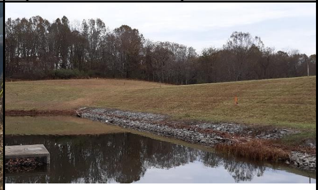
Image 6: Riprap on upstream slope
