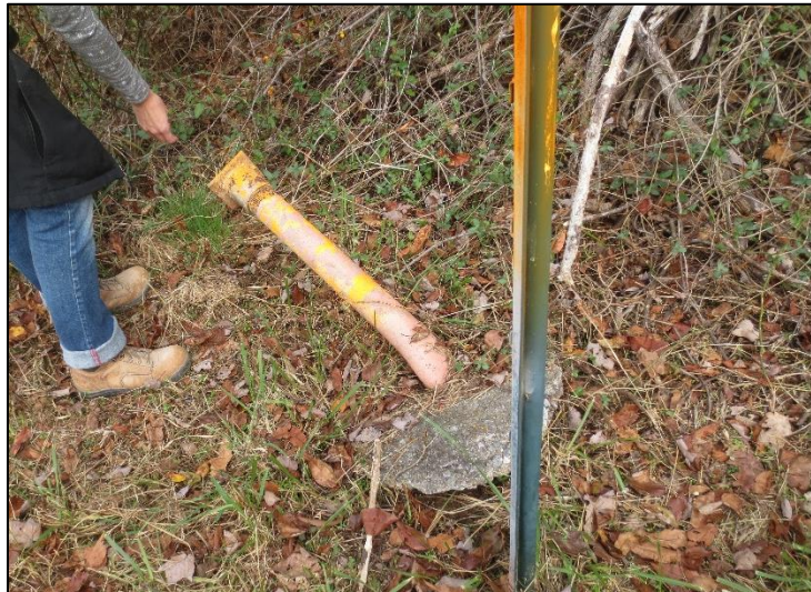
Photograph 11: Damage to observation well #11.
