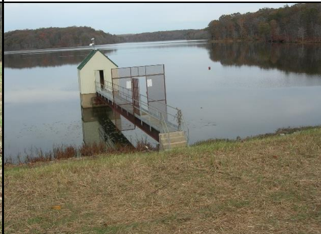
Image 42: Water intake structure
