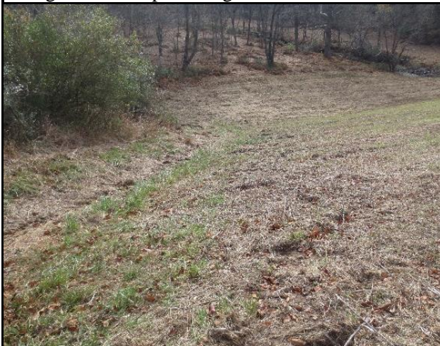
Image 15: Left downstream groin. Note rutting
