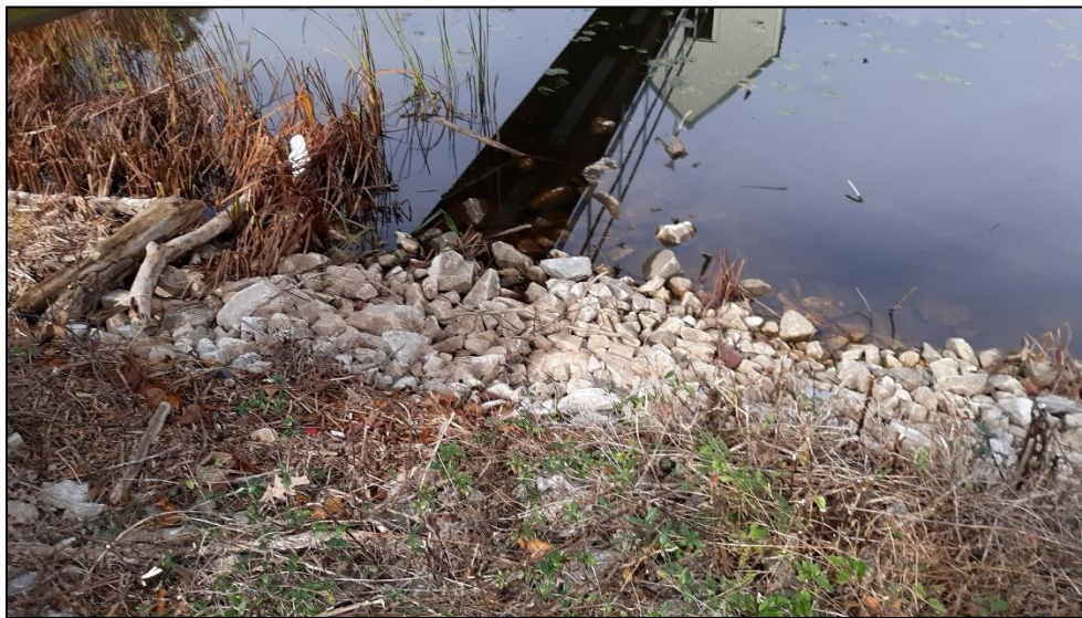
Photograph 9: Reservoir upstream slope riprap and debris.
