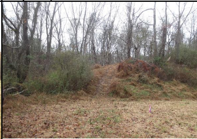
Image 40: ASW outside slope at outlet. Note path which leads to electrical standpipe and fourteenth observation well
