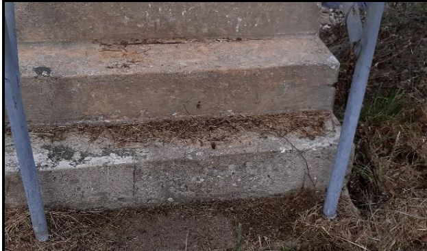
Image 47: Stairway to water intake tower catwalk. Note deterioration in concrete
