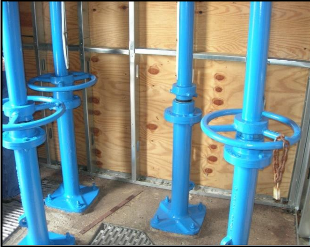
Image 49: Inside water intake structure, intake slide gate operators on right side. Note broken operator handle
