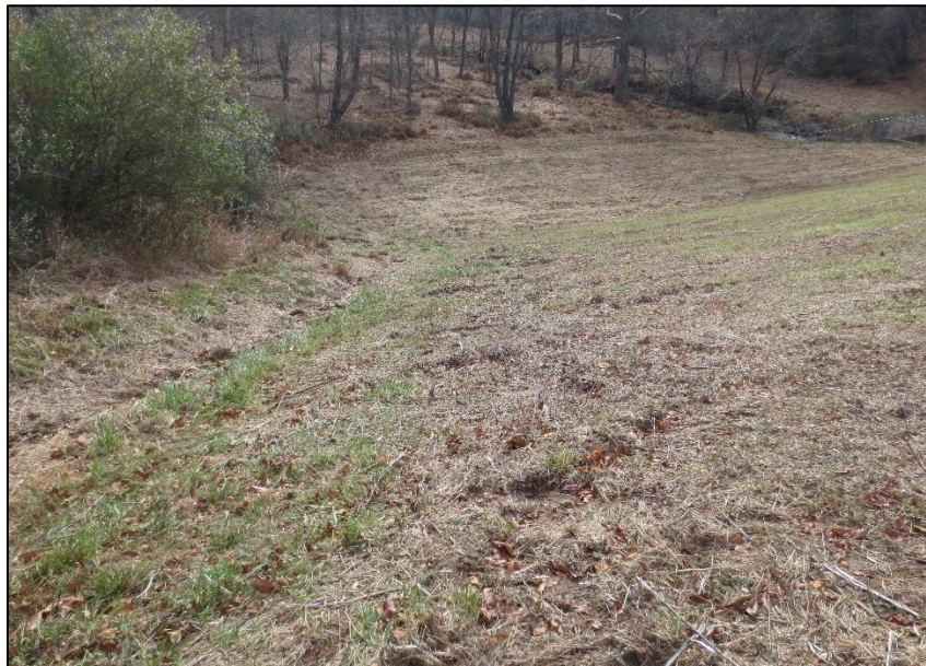
Photograph 4: Disturbance of left downstream slope, likely by grass cutting equipment.
