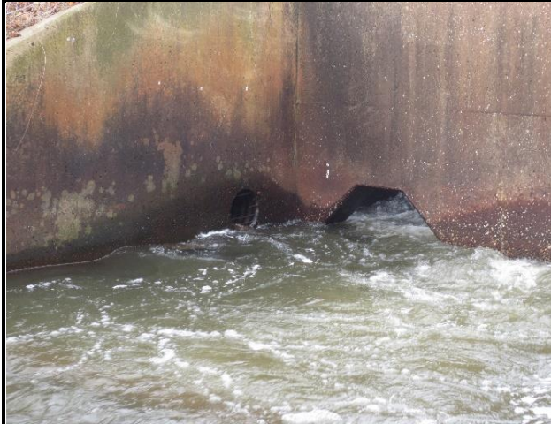
Image 23: Right toe drain outlet at impact basin
