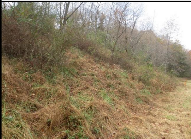
Image 39: ASW outside slope, downstream
