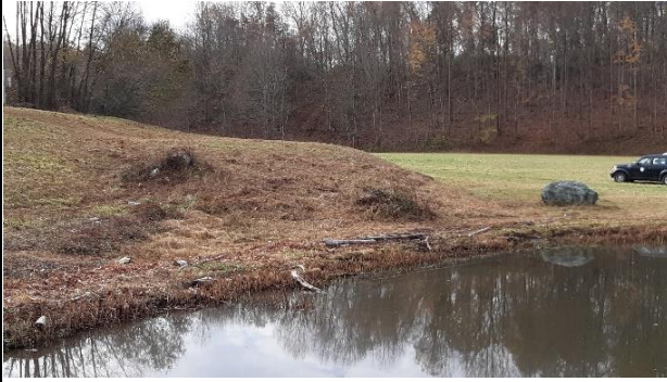
Image 31: Training dike. Note woody debris
