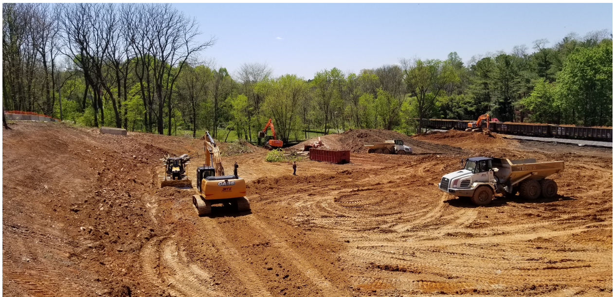
Langdon stormwater facility site, Westminster
