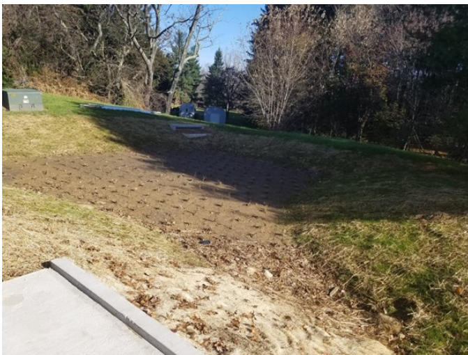
Bio-Retention Facility installed at the end of McAllister Lane
