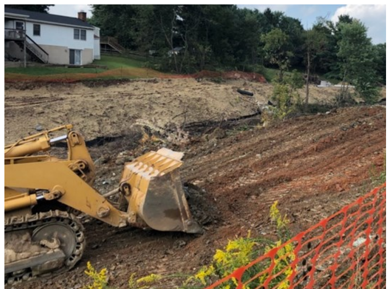
grading the slope along Ridge Avenue
