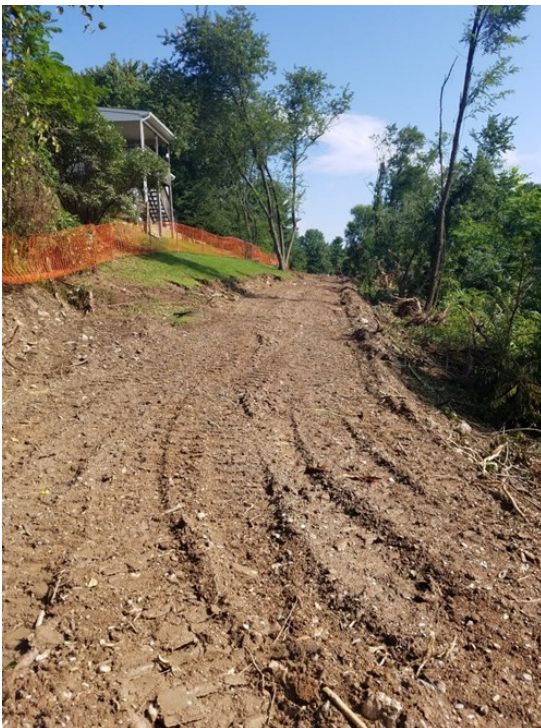
clearing for the sewer replacement
