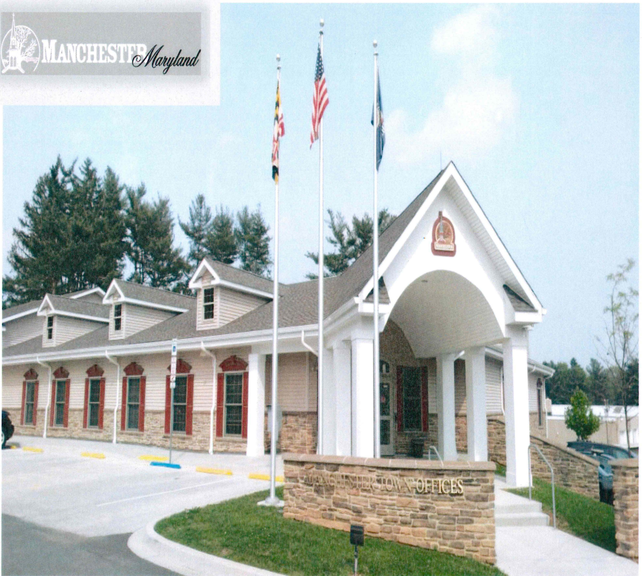
Manchester Town Offices and Police Station
