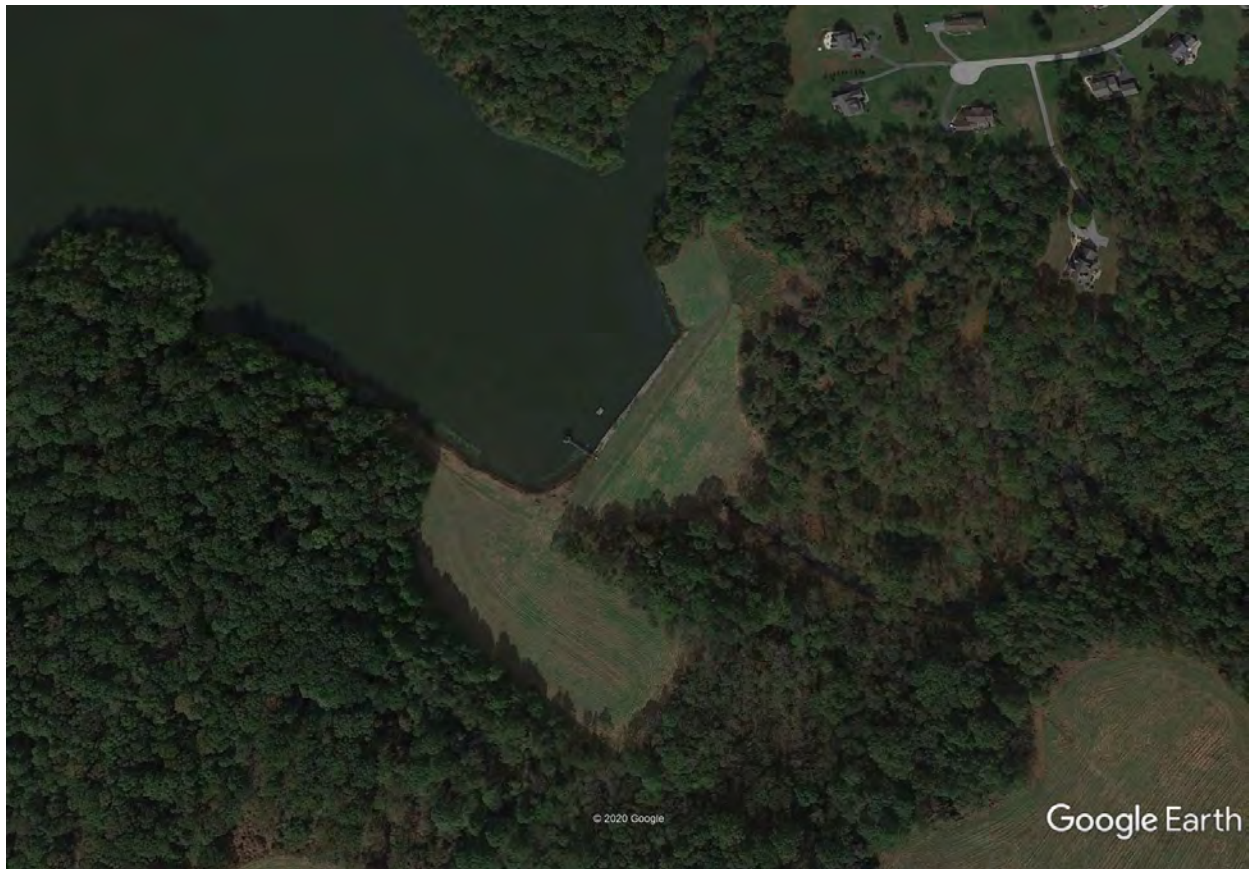
Figure 1: Piney Run Dam aerial photograph
