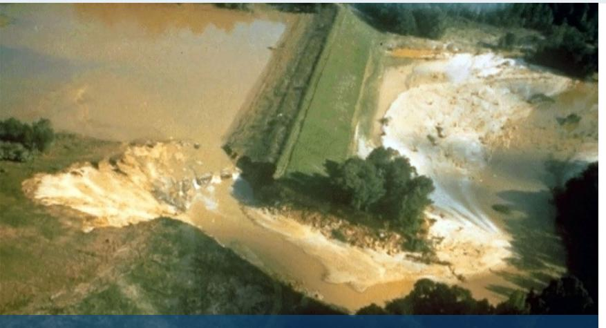
Black Creek Site 53 (MS) failure from spillway erosion in 1983 (courtesy: NRCS)
