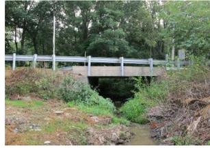
This project provides funding to replace the small bridge, located in western Carroll County near the Town of New Windsor. The existing structure is concrete encased steel beams on stone masonry abutments. The type of replacement structure will be determined based on an alternatives analysis. The structure width and waterway opening will be evaluated as part of the analysis. The structure is posted for weight limits.
