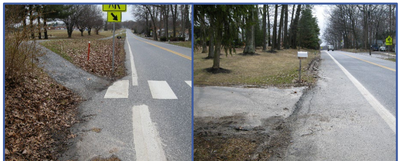
Above Left: crosswalk and walking path at Johnsville Rd & Victor Dr Above Right: northbound Johnsville Rd, looking towards Eldersburg ES
