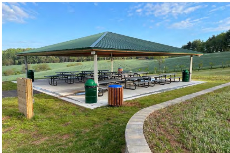
FIGURE 1: BEAR BRANCH PAVILION
