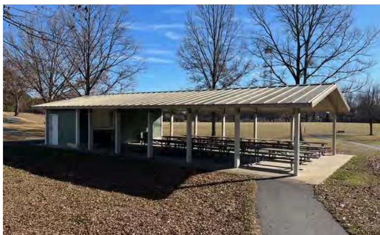
FIGURE 6: SANDYMOUNT PARK PAVILION
