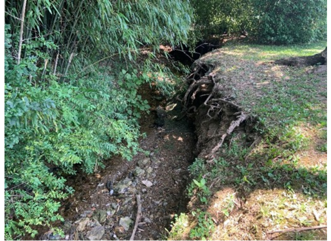
Hampstead Valley 4 Restoration
