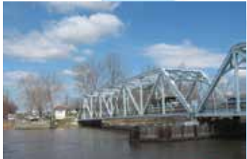
MD 331, Dover Bridge replacement
