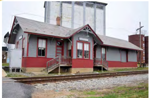
Hampstead, MD train station now
