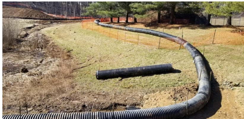
The clean water diversion being installed at the Oklahoma Phase IV facility.
