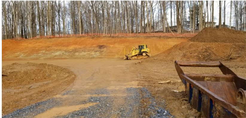
Excavation and hauling of excess material.
