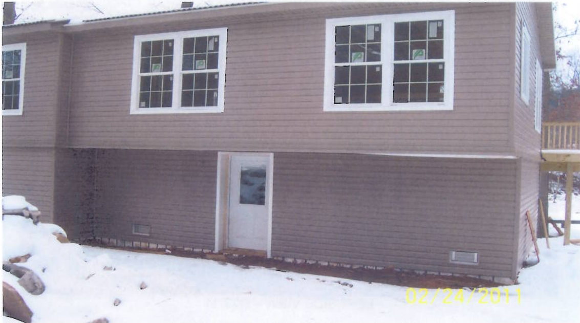
FRONT-RIGHT CORNER VIEW – 2/24/11
