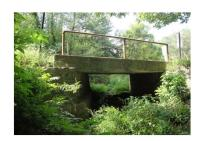
This project provides planned funding to replace the small bridge, located in western Carroll County near the Town of New Windsor. The existing structure is concrete encased steel beams on stone masonry abutments. The type of structure will be determined based on an alternatives analysis. The structure width and waterway opening will be evaluated as part of the analysis.
