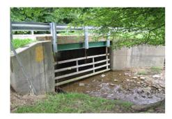
This project provides funding to replace the existing bridge located at the intersection of Cape Horn Road and Harvey Gummel Road. The existing structure is a steel beam bridge on concrete abutments. The new structure will be determined based on an alternatives analysis.
