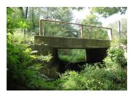
This project provides planned funding to replace the existing small bridge, located in western Carroll County near the Town of New Windsor. The existing structure is constructed of concrete encased steel beams on stone masonry abutments. The type of structure will be determined based on an alternatives analysis. The structure width and waterway opening will be evaluated as part of the analysis.
