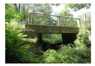
This project provides planned funding to replace the existing small bridge, located in western Carroll County near the Town of New Windsor. The existing structure is constructed of concrete encased steel beams on stone masonry abutments. The type of structure will be determined based on an alternatives analysis. The structure width and waterway opening will be evaluated as part of the analysis.
