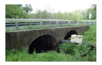
This project provides funding to replace the existing two cell culvert, located east of Union Mills, with a new structure.
