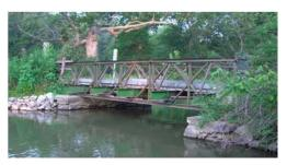
This project provides funding to replace the acrow panel bridge, located in northern Carroll County, with a new structure.
