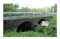
This project provides funding to replace the existing two cell culvert, located east of Union Mills, with a new structure.
