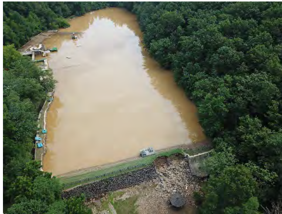
Cascade Lake Dam failure, July 2018 (Carroll County Government photo)
