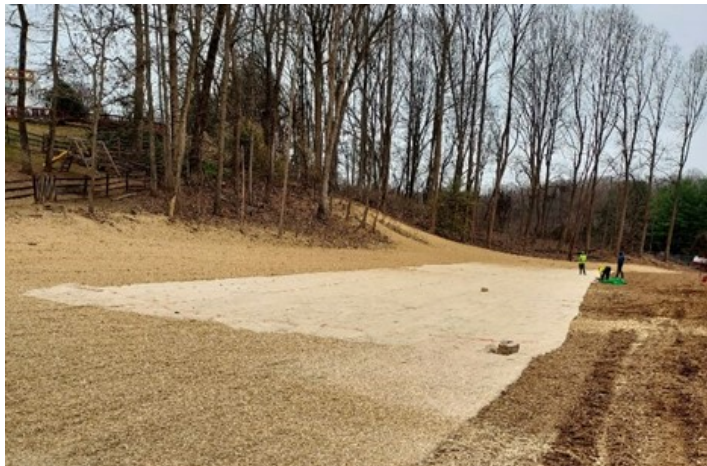
New graded and stabilized swale at Oklahoma awaiting turf growth
