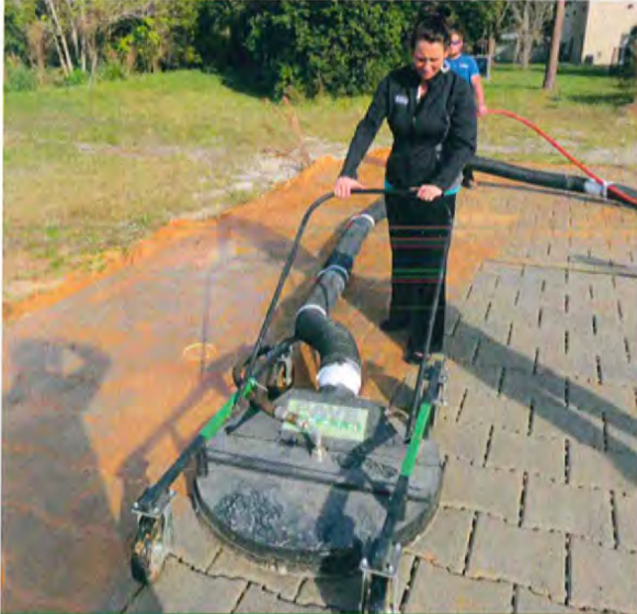
Smaller Sites: PaveDrain Vac Head
