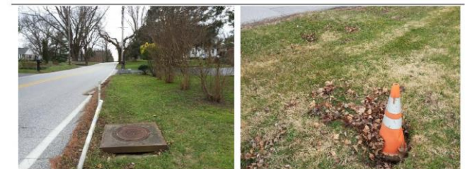
Figure 1: Opportunity to improve existing conveyance system.
