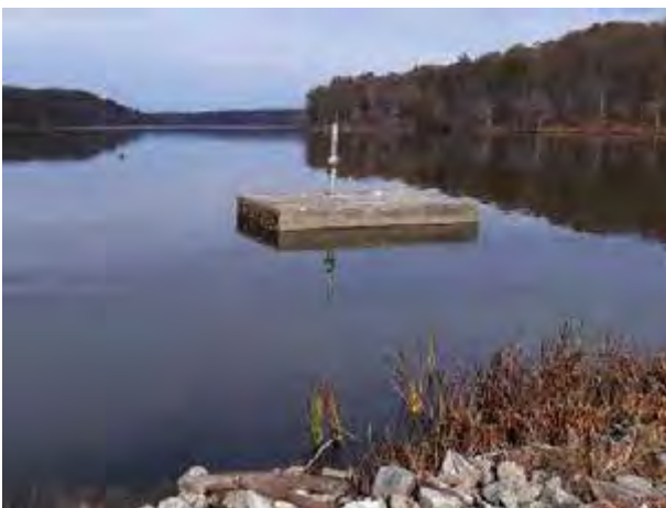
Above-water portion of riser
