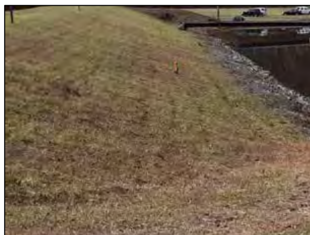
Upstream embankment slope and wave protection.
